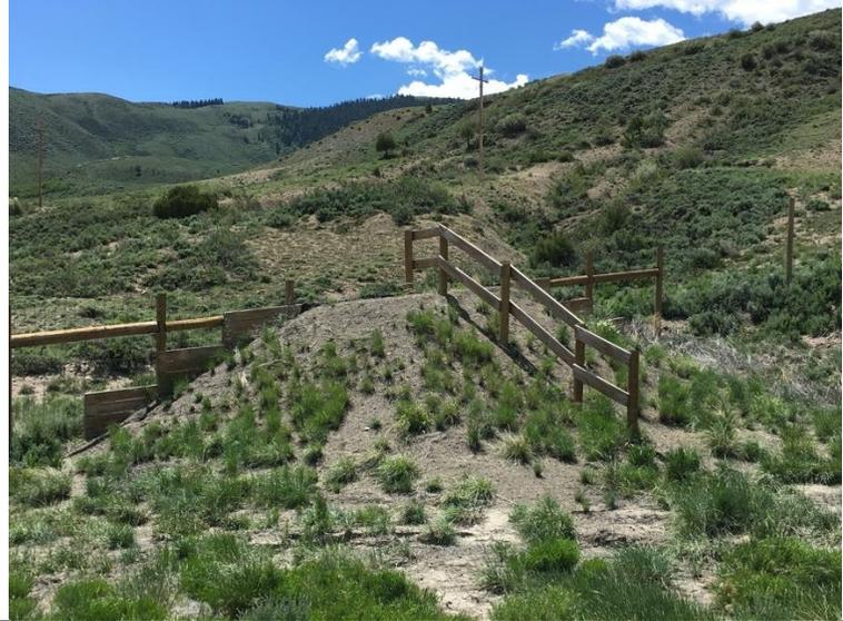
Escape Ramp – 3:1 slope without perpendicular rail fence
