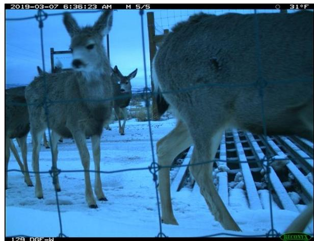
Figure 5-2. Mule deer breaching a wildlife guard by walking on snow packed in between the bars.
