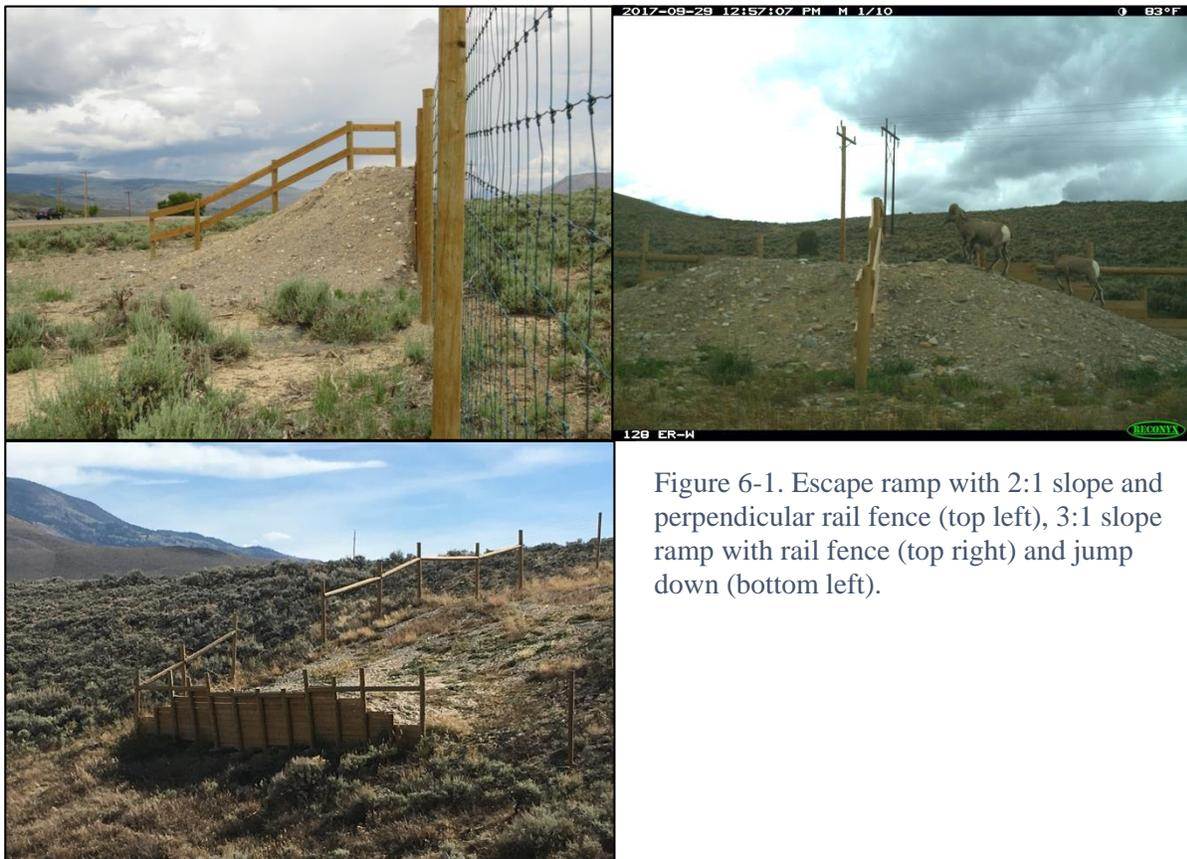
Figure 6-1. Escape ramp with 2:1 slope and perpendicular rail fence (top left), 3:1 slope ramp with rail fence (top right) and jump down (bottom left).
