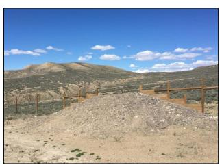
*Figure 30.* Example of an escape ramp with a 2:1 slope with perpendicular rail fence (left) and a ramp with a 3:1 slope with no rail fence (right).
