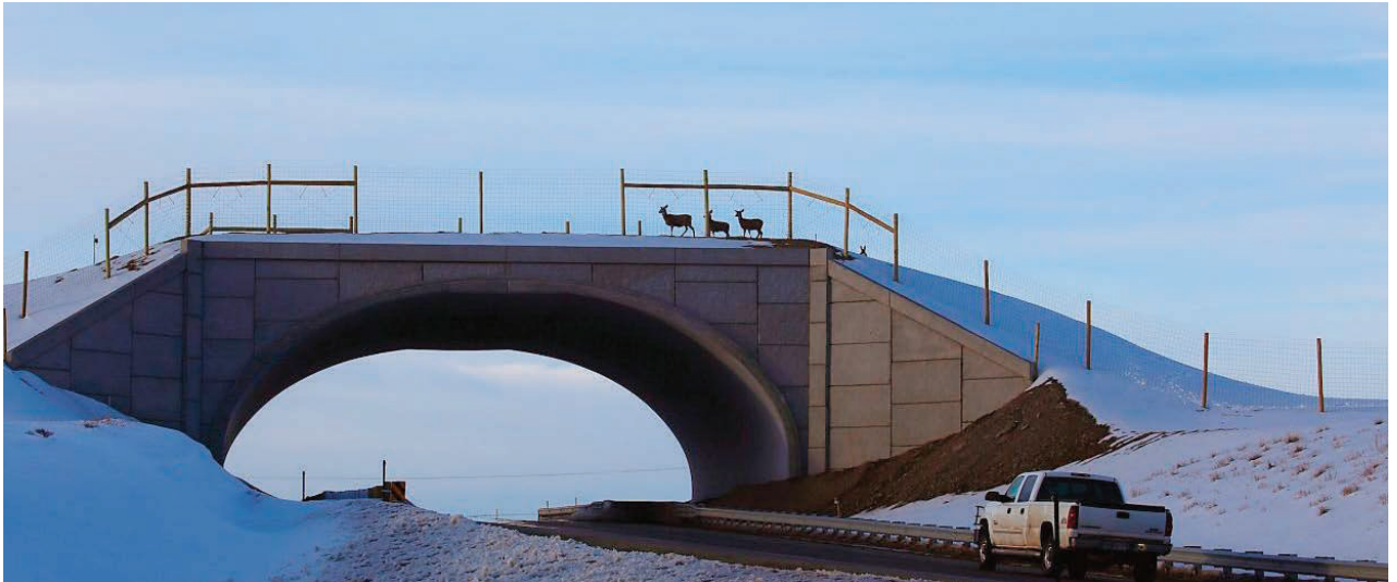
ABOVE AND BEYOND —Colorado Highway 9 has long been a slaughterhouse for elk and mule deer, but wildlife overpasses and underpasses have cut wildlife collisions by 90 percent.
