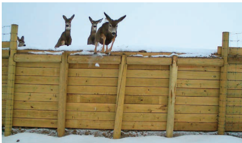
JUMP TO SAFETY —Tall fences keep wildlife off the highway and steer them to overpasses and underpasses, but if animals do get on the road, jump-out ramps allow a quick escape.
