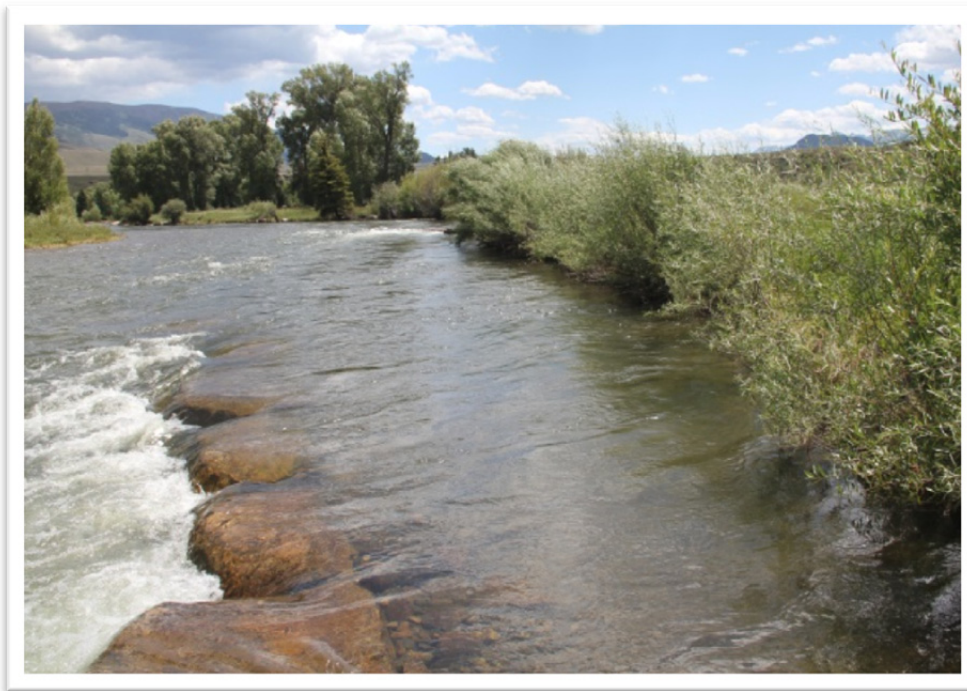
Figure 17. Post-restoration view of a J-Hook Vane installed on the Blue River near same location as Figure 16 on the Blue Valley Ranch (note same cottonwood gallery). The right bank with abundant willows was previously an actively eroding bank without vegetation; photo taken looking upstream.
