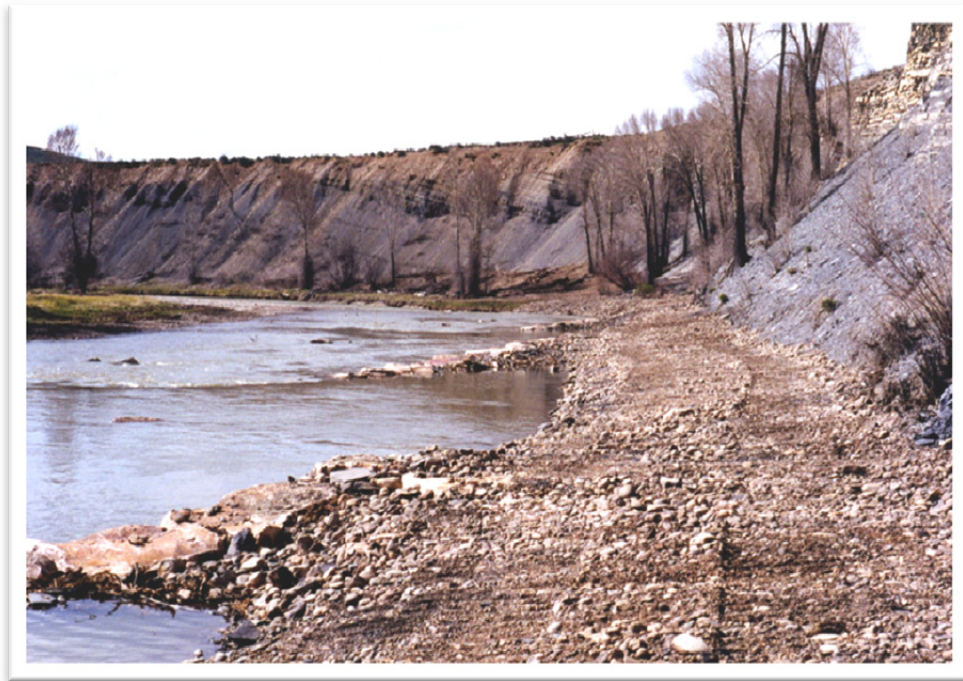
Figure 18. A J-Hook Vane and a bankfull bench shown immediately following construction on the Blue River. Willow or cottonwood transplants were not placed on the bench as the decision was made to let the river do it.
