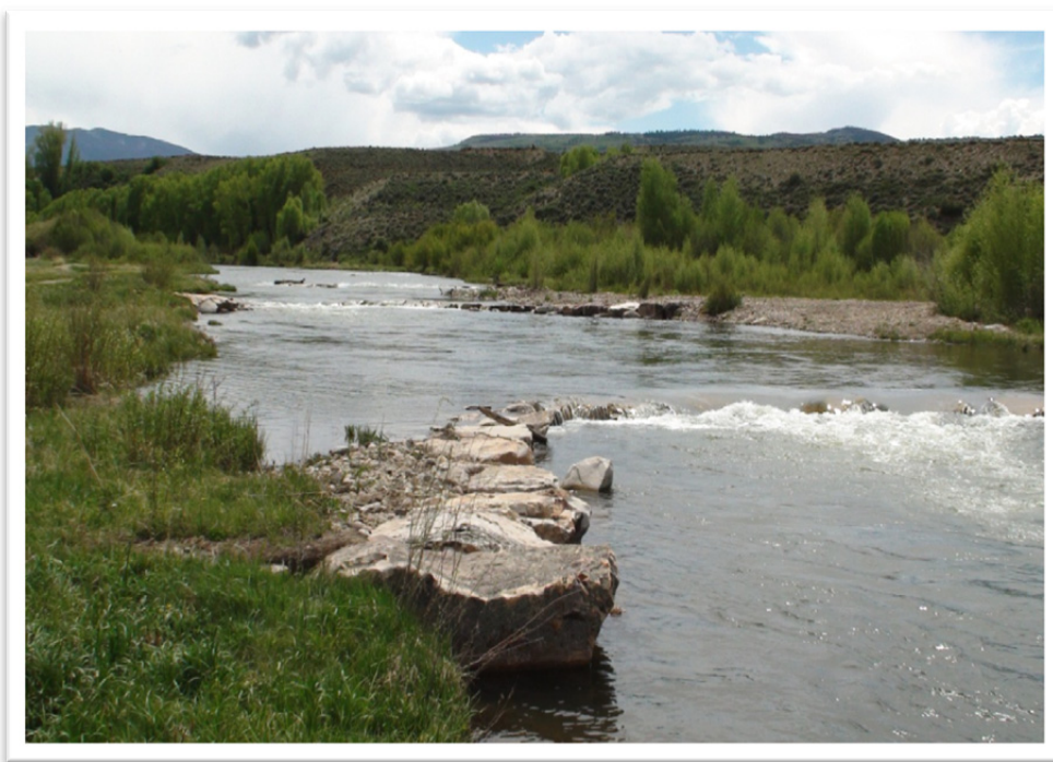
Figure 24. A Cross-Vane structure constructed on the Blue River. Note the low gradient and low velocity stage of the river upstream of vane arm.
