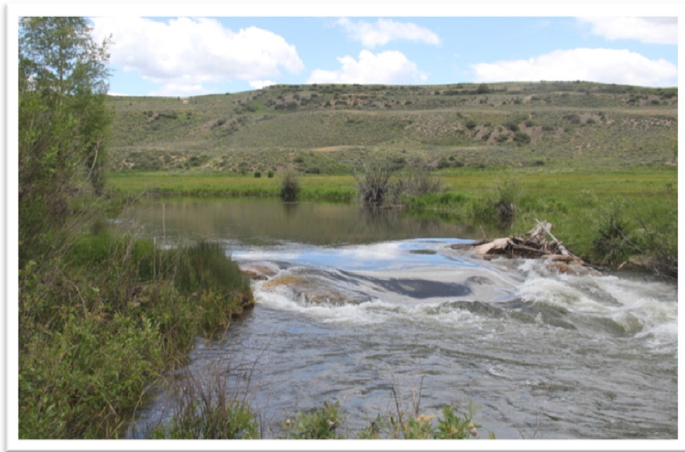
Figure 30. Oxbow with step-pool outlet, showing the flat slope of the oxbow channel above the step-pool outlet.
