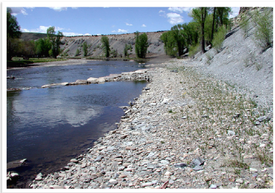
Figure 19. Same location as in Figure 18 one year post-construction and following a flood that deposited fine sediment and cottonwood seedlings on the bankfull bench.
