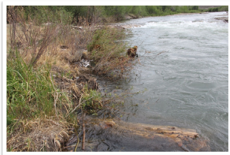
Figure 12. Toe wood below a J-Hook Vane on the main Blue River on the Blue Valley Ranch that was installed to provide a natural appearing structure, reduce streambank erosion, and provide holding cover for fish.
