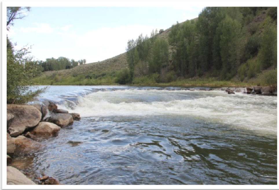
Figure 23. A Cross-Vane structure used for a flow diversion on the Blue River shown during a high flow period. This structure is proposed for the boating ramp location because of the lower velocity and higher stage upstream of the vane arm.
