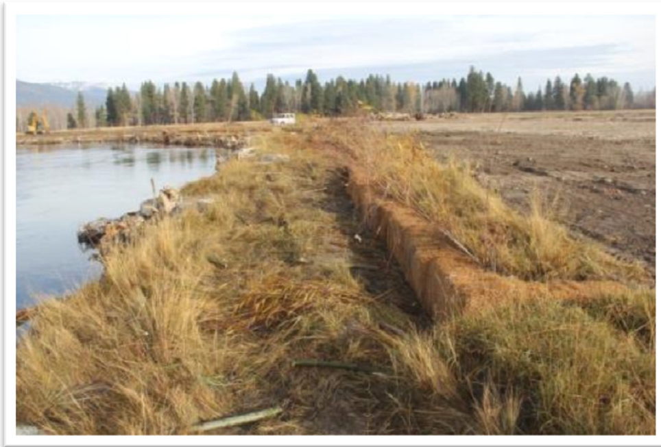
Figure 13. The use of hay bales and willow cuttings on the upper one-third of a Toe Wood bank on the Bitterroot River, Montana. The bankfull stage maximum pool depth is 18 ft at this location.
