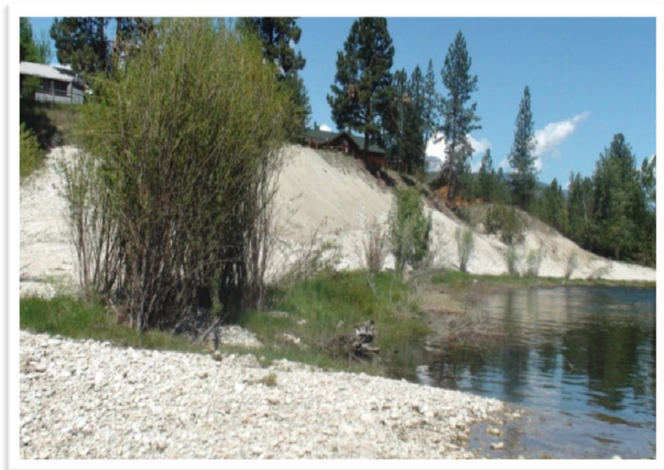
Figure 14. Toe Wood and a constructed bankfull bench against a high eroding terrace bank, Bitterroot River, Montana. The maximum pool depth is 20 ft along this meander bend. The submerged wood has stayed in place throughout four extreme flood events occurring since implementation.
