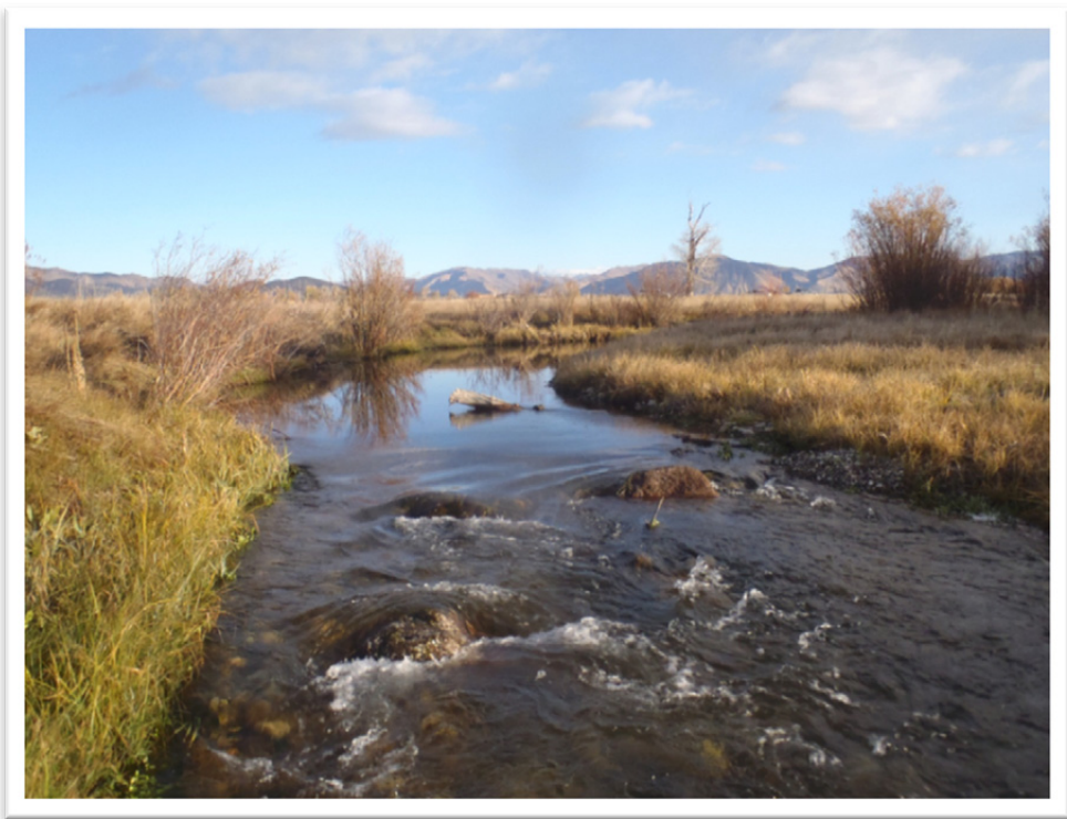
Figure 26. Converging Rock Clusters installed on Crystal Creek, Heartrock Ranch, Idaho.
