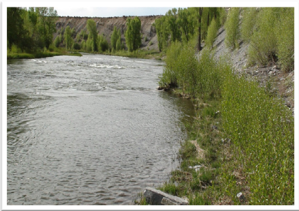
Figure 20. Same location as Figure 18 five years post-construction, showing the establishment of a new cottonwood gallery and a functioning bankfull bench.
