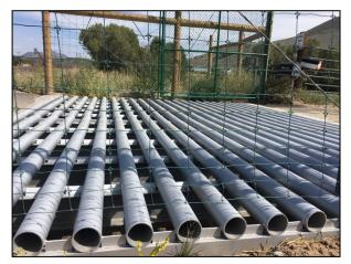
*Figure 16.* Round bar deer guard design installed at select locations during Phase 2 construction.
