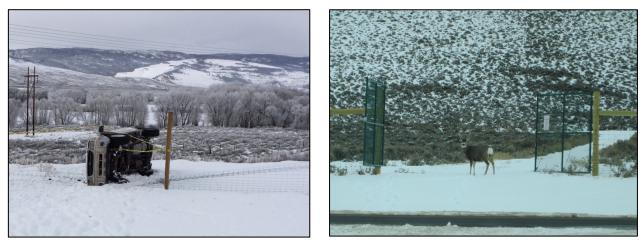
*Figure 33. a*) Gap in wildlife exclusion fence due to a vehicle that ran off the road (left). *b*) Mule deer exiting through a swing gate left open by CPW to allow the animal to safely exit the fenced right-of-way under their supervision (right).
