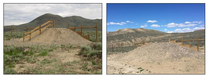
*Figure 17.* Examples of escape ramp with 2:1 slope and rail fence (left) and 3:1 slope with no rail fence (right).
